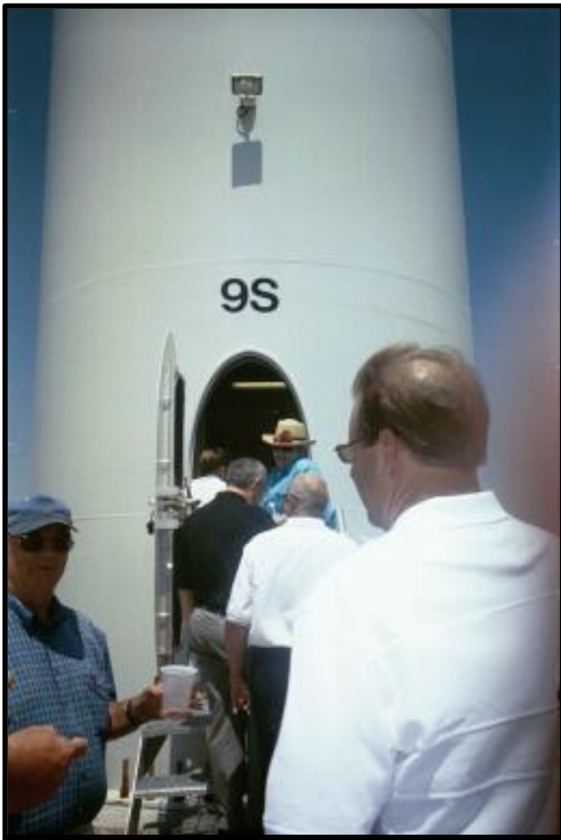
Above: Dedication attendees check out the inside of one of the GE 1.5 MW turbines.
