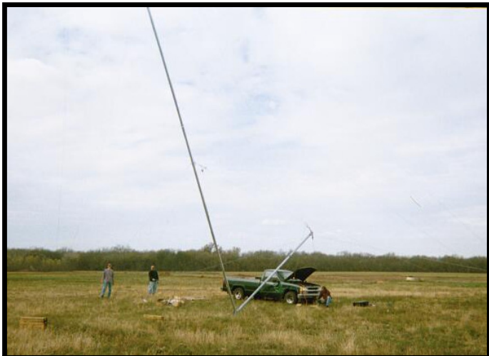
Tower raised with battery-powered winch.
